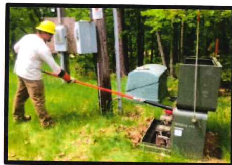
Linemen need room to work
